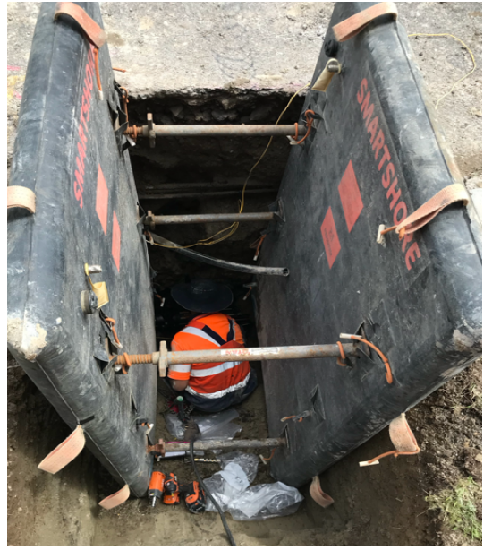
Trench Shield Protection of worker
